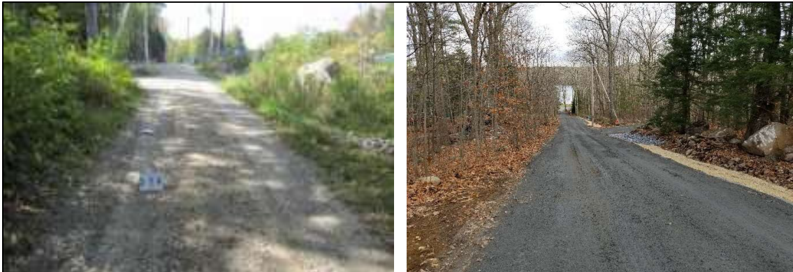
Before and After Photos - Camp Tracy road project
