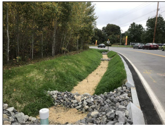
After: Underdrain soil filters installed on Morin Street
