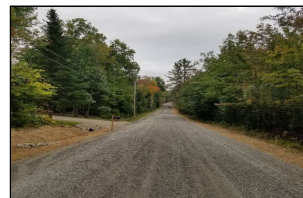
Bacon Road (Mercer) after crowning and ditch stabilization
