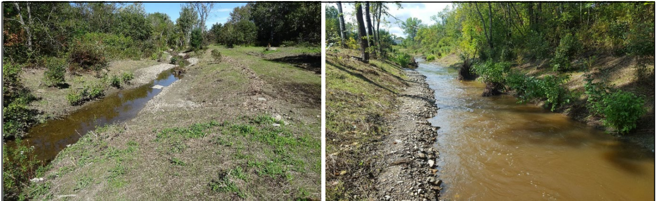
Instream restoration work included adding gravel bars, root wads and plantings along 550 feet of stream.
