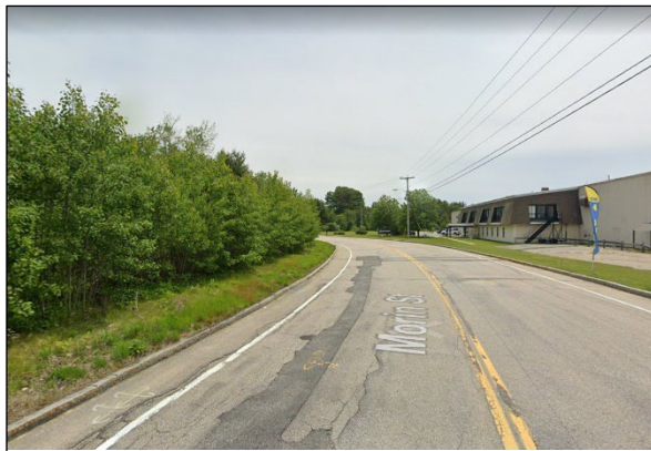
Before: Morin St before BMP installation
